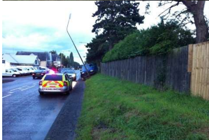
Outside 29 Cambridge Road - July 2012
